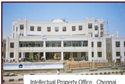
Intellectual Property Office, Chennai
